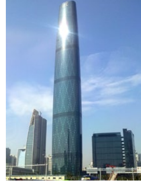
Building Height: 1,493 ft Diagrid Type: AESS Architect: Wilkinson Eyre Engineer: Arup Photograph © 慕尼黑啤酒 via Wikimedia Commons
