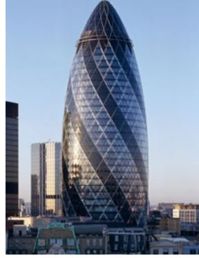
Building Height: 590 ft Diagrid Type: Concealed Architect: Foster + Partners Engineer: Arup Photograph © Swiss Re
