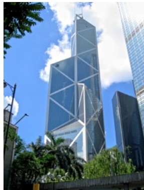
Building Height: 1,205 ft Diagrid Type: Diagonalized Core Architect: I. M. Pei Engineer: Leslie E. Robertson Associates Photograph © WiNG via Wikimedia Commons
