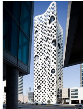
Building Height: 374 ft Diagrid Type: Concrete Diagrid Variation Architect: RUR Architecture Engineer: Ysrael A. Seinuk Photograph © Nelson Garrido
