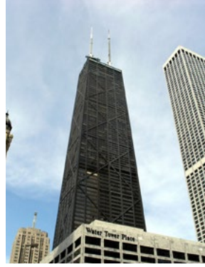
Building Height: 1,128 ft Diagrid Type: Diagonalized Core Architect: SOM Engineer: SOM Photograph © Chicago Architecture Foundation
