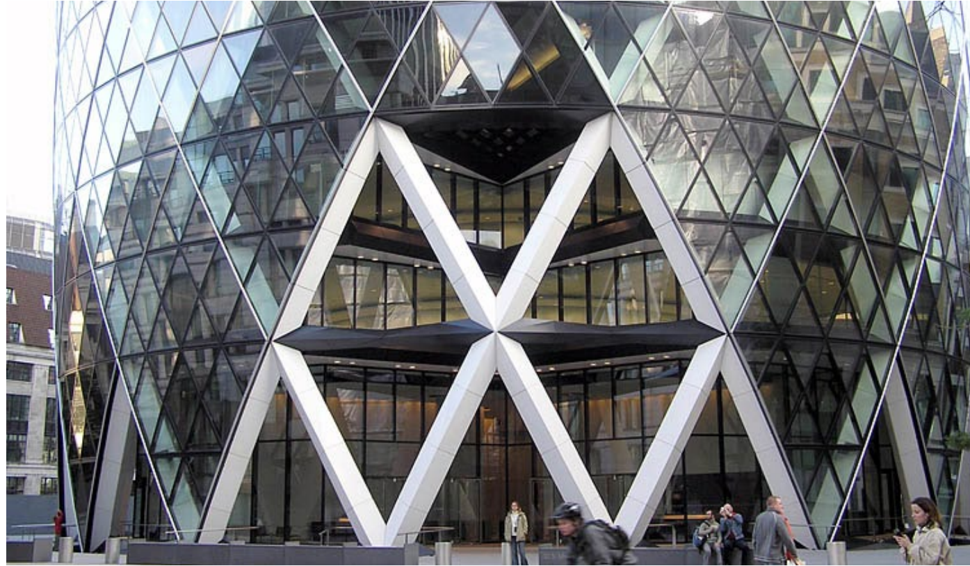
Swiss RE Building (30 St. Mary Axe), London, England. Foster + Partners, 2003. Photograph © Adrian Pingstone via Wikimedia Commons, 2004.
