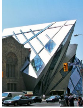
Building Height: 6 floors Diagrid Type: Concealed Architect: Libeskind w/ Bregmann and Hamman Engineer: Arup Photograph © Aviad2001 via Wikimedia Commons
