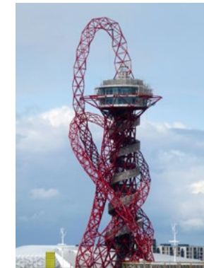
Building Height: 377 ft Diagrid Type: AESS Architect: Anish Kapoor, Cecil Balmond Engineer: Arup Photograph © Cmglee via Wikimedia Commons
