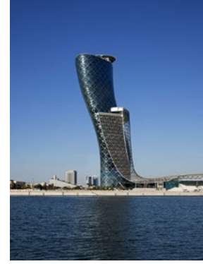
Building Height: 540 ft Diagrid Type: AESS Architect: RMJM Engineer: RMJM Photograph © Graitect
