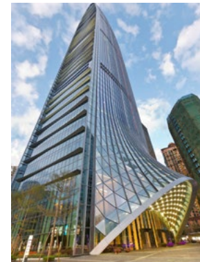
Building Height: 1,499 ft Diagrid Type: Diagonalized Core Architect: TFP Architects Engineer: SOM Photograph © Carsten Schael
