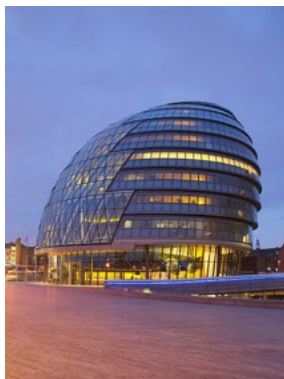
Building Height: 10 floors Diagrid Type: AESS Diagrid to Support Glazing Architect: Foster + Partners Engineer: Arup Photograph © MatthiasKabel via Wikimedia Commons
