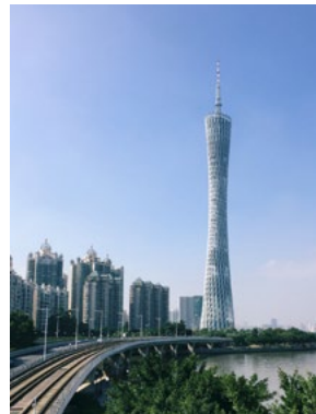
Building Height: 1,969 ft Diagrid Type: External AESS Diagrid Architect: Mark Hemel / Barbara Kuit / IBA Engineer: Arup Photograph © Unsplash/Lycheeart
