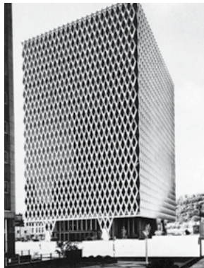
Building Height: 13 floors Diagrid Type: Concealed Architect: Curtis and Davis Engineer: Leslie E. Robertson Associates Photograph via Pittsburgh-Post Gazette
