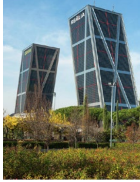
Building Height: 374 ft Diagrid Type: Diagonalized Core Architect: Johnson / Burgee Engineer: Leslie E. Robertson Associates Photograph © Andrew Michael, 2016
